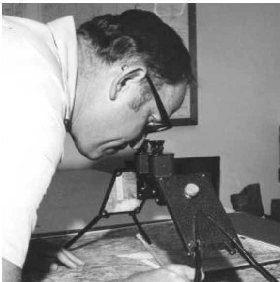
Loyal Quandt using a “stereoscope” to evaluate landscapes and match joins between soil maps. Lancaster County, 1973.
