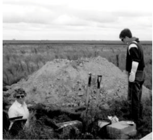
L-R: Maurice Mausbach, NRCS, and Mark Kuzila, Conservation and Survey Division, collecting Holdrege soil samples for laboratory analysis. Phelps County, 1980's.
