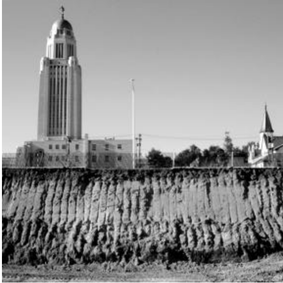
State Capitol of Nebraska in Lincoln. Excavation for building in foreground.
