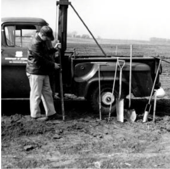
Dean DaMoude displaying power probe tube, hand probe, spade, shovel, and hand auger. Cuming County, 1957.
