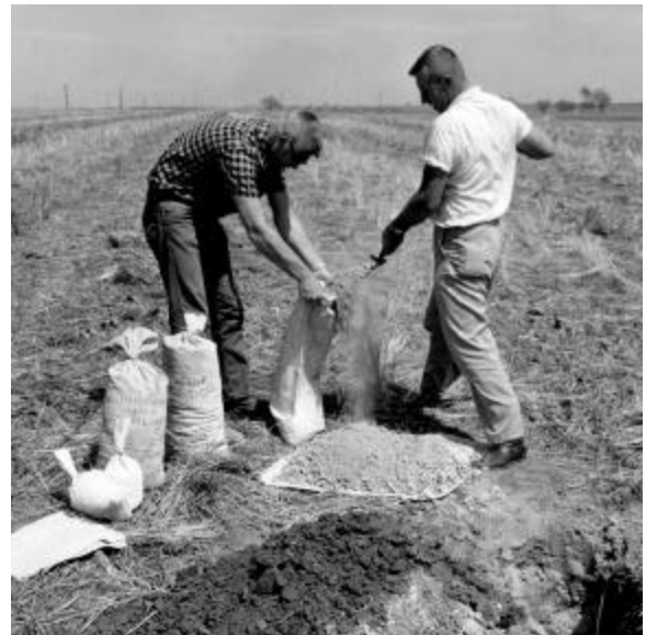
Soil scientists collecting soil samples for engineering soil tests. Western Nebraska, 1962.
