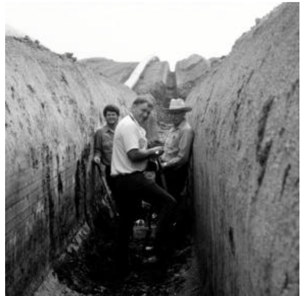
L-R: Charles Morris, Dave Lewis, and John Elder examining soils in Pathfinder pipe-line trench. Fillmore County, 1982.
