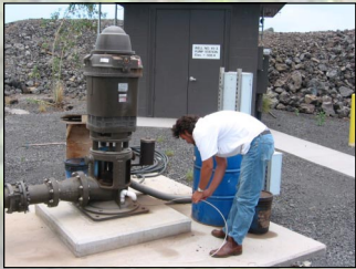
Inspecting municipal well, Kona, Hawai'i
