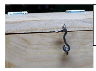
Drill a pilot hole and attach the "hook" portion of the hookand-eyelet. Should have a "snug" fit.
