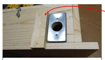
Add the cleat below the metal plate. Glue and nail/screw. Be sure the screw/nail here is short enough that it does not penetrate the wood.
