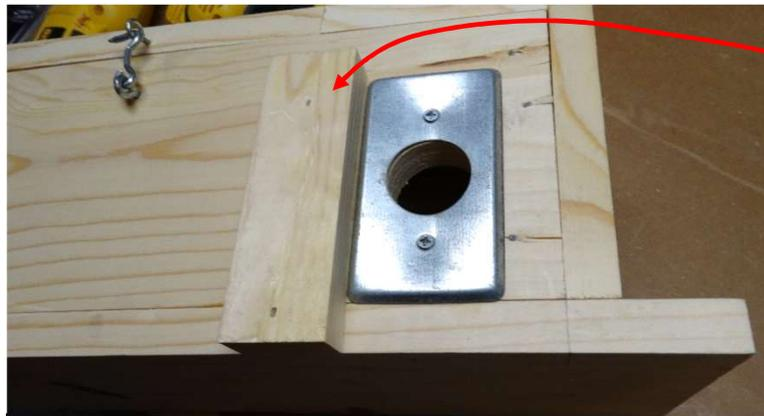
Add the cleat below the metal plate. Glue and nail/screw. Be sure the screw/nail here is short enough that it does not penetrate the wood.
