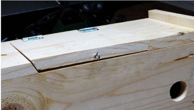
Drill a pilot hole and attach the “eyelet” portion of the hook-and-eyelet.
